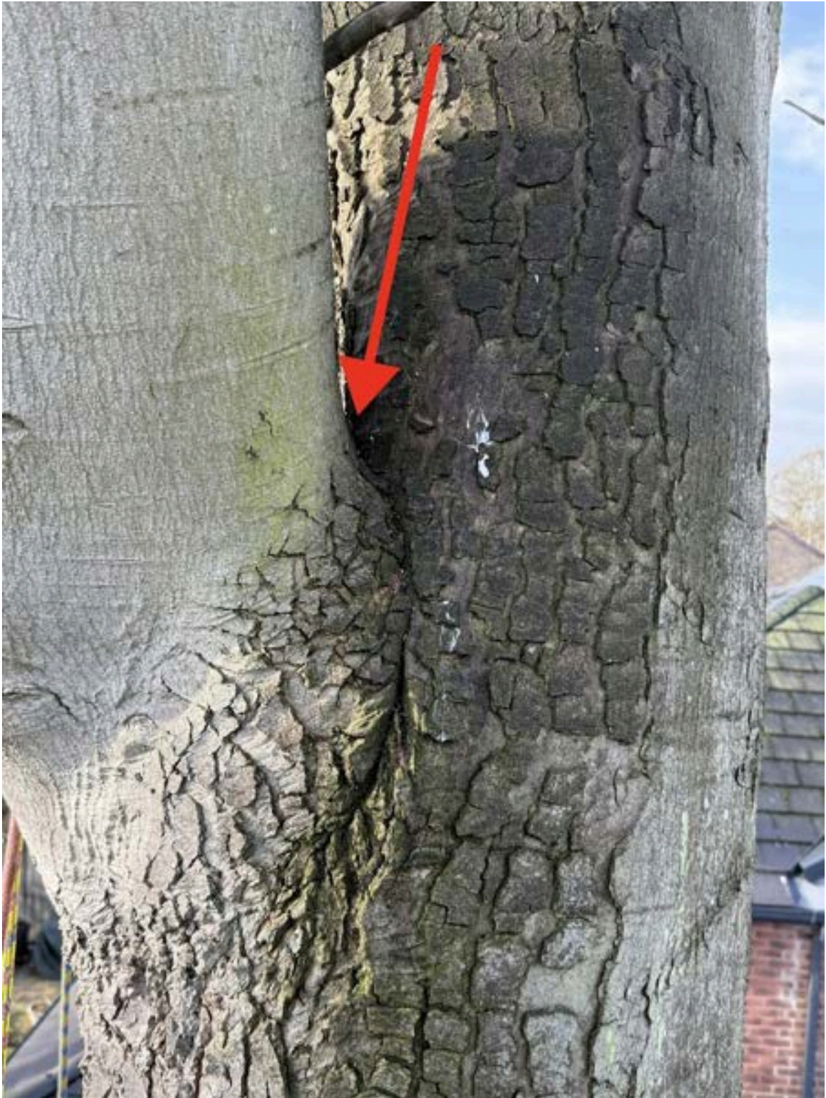
This is another potential point of failure.
